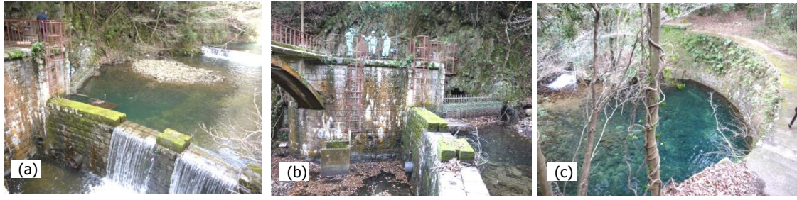
Fig. 8: Nunobiki Separation dam (a), Intake (b) and Shut up dam(c)
