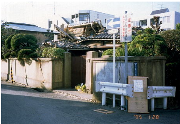
Photo 1 A collapsed wooden house (originally 2-storied) in Higashinada-Ward 11 days after the 1995 Hyogo-ken Nanbu (Kobe) earthquake (Photo by H. Kawase).
