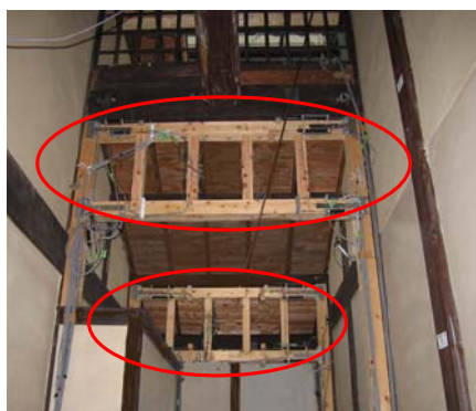
Photo 6 Seismic reinforcement using laddery frames
