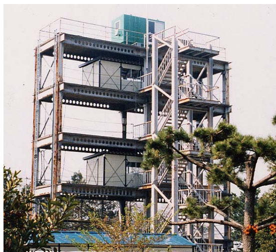
Photo 2 Full-scale five-story steel building
