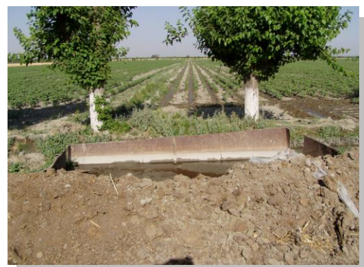
Fig.4 Settling construction for semi-liquid manure removal into the irrigated drylands
