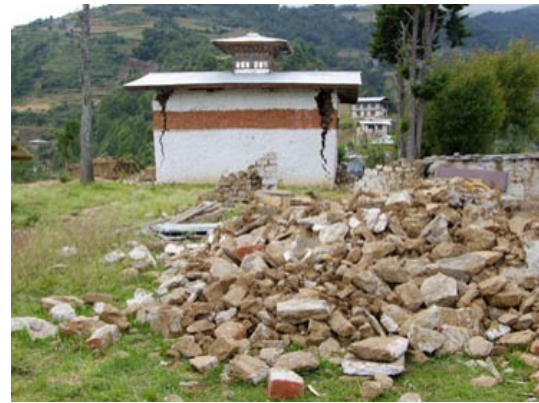
Photo 1a Collapsed house by 2009 earthquake in Trashingang (eastern Bhutan) (Komori, J., Pers. Comm.).
