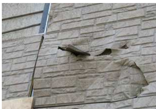
g. Roof tile stuck into a wall
