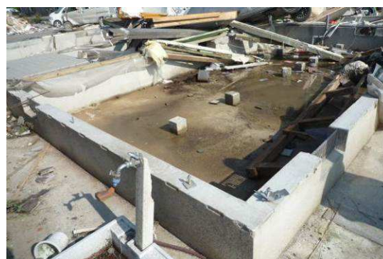
Fig. 7 Foundation of blown off wooden house ( quote from the report of KAKENHI, 2013 )
