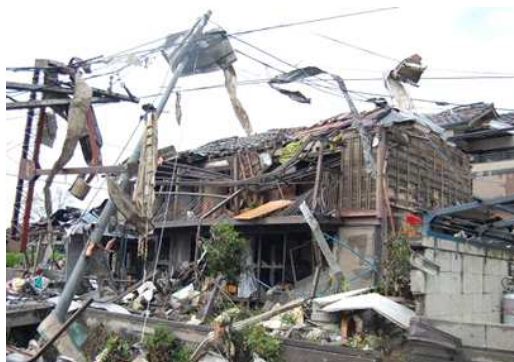
a. Flying debris twining around power lines
