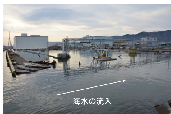
Figure 7 Invasion of seawater into the harbor, Ishinomaki fishery port.
