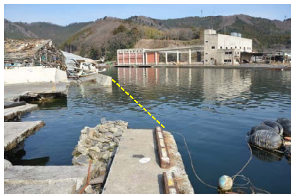
Figure 10 Lost sea walls in Onagawa fishery port.
