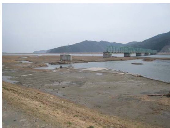
Figure 12 View of the Shin Kitakami bridge.
