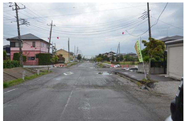
Figure 24 Ground deformation in Hinode cho, Itako city.
