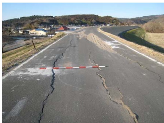
Figure 18 Longitudinal cracks at the top of the embankment of the Kitakami River (45.5k).
