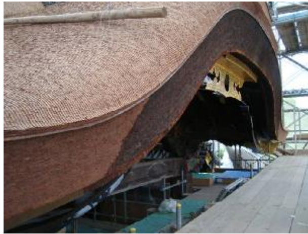
Fig. 4 Kyoto. The restoration site of the Imperial gateway in Nijo Castle. June 25, 2013 Detail of the kara-hafu . The dark area does not restored. (2013 © Olimpia Niglio)
