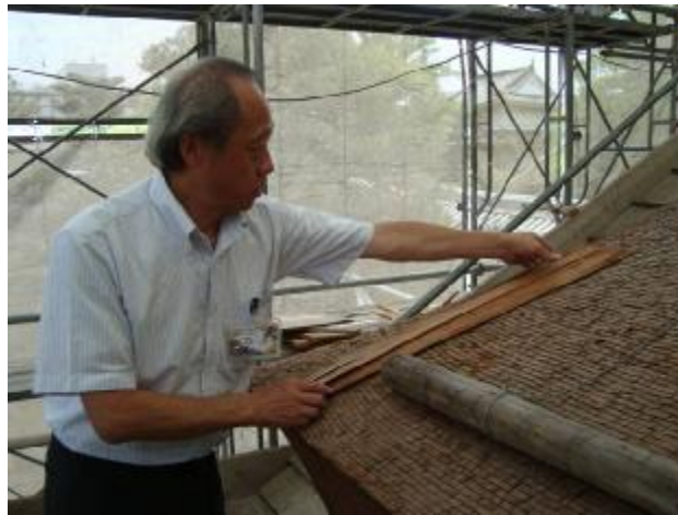
Fig. 5 Kyoto. The restoration site of the Imperial gateway in Nijo Castle. June 25, 2013 The Architect Goto describes the restoration of roof with bark of the cypress. (2013 © Olimpia Niglio)
