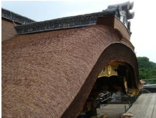
Fig. 6 Kyoto. The restoration site of the Imperial gateway in Nijo Castle. July 30, 2013 Detail of the kara-hafu after the restoration (2013 © Olimpia Niglio)
