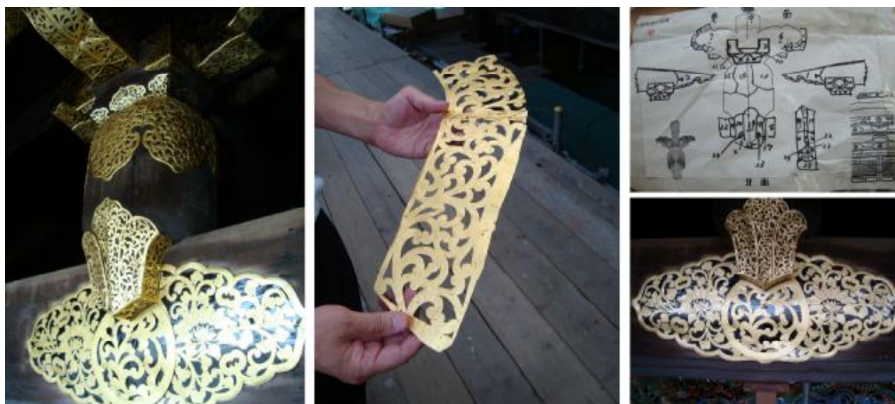
Fig. 3 Kyoto. The restoration site of the Imperial gateway in Nijo Castle. June 25, 2013 Details of the copper and gold decorations, during restoration. (2013 © Olimpia Niglio)
