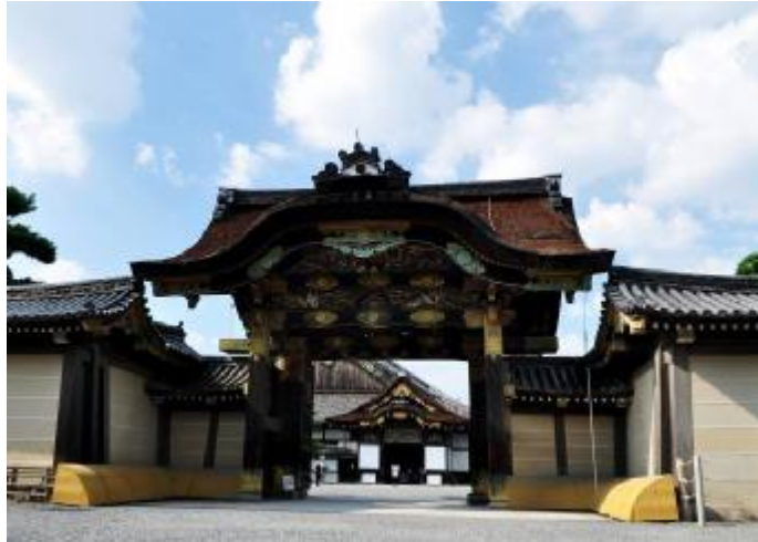
Fig. 1 Kyoto. The Imperial Gateway in Nijo Castle before the restoration (2008 © Olimpia Niglio)
