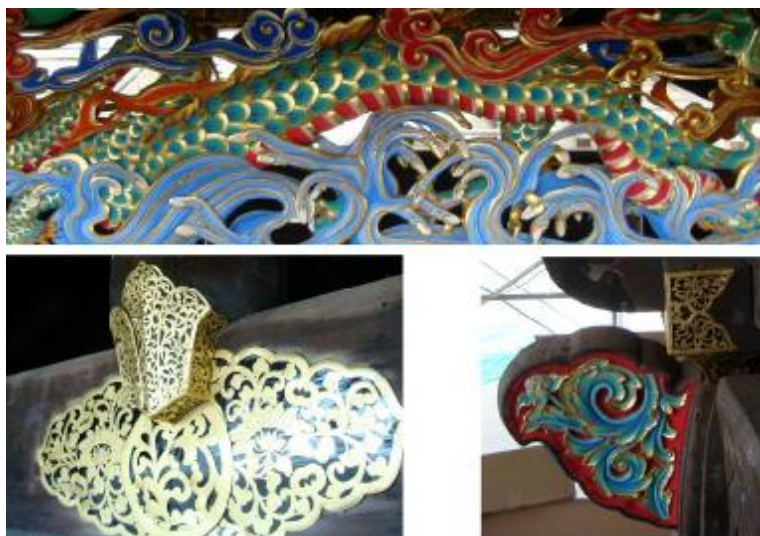
Fig. 2 Kyoto. The restoration site of the Imperial gateway in Nijo Castle. June 25, 2013 Details of the bas-reliefs in wood and of the decorations with typical colors, during restoration. (2013 © Olimpia Niglio)
