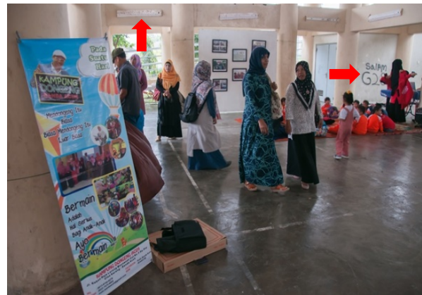
Figure 5.32 Vandalism on the escape building
