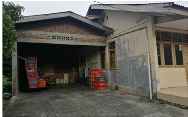
Figure 4.19 Storage area (extension)
