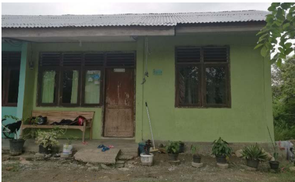
Figure 5.19 House constructed by World Vision
