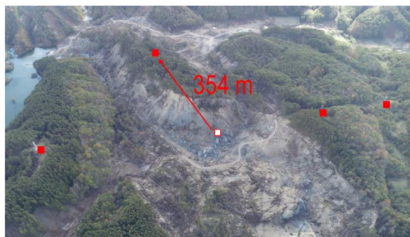
Photo 10 Large-scale landslide on Hidaka-Horonai area. ■: Power tower; □: Former location of power tower (taken on October 18, 2018)
