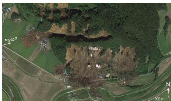
Photo 6 Landslides on Tomisato area (After Google earth, photo of September 11, 2018)
