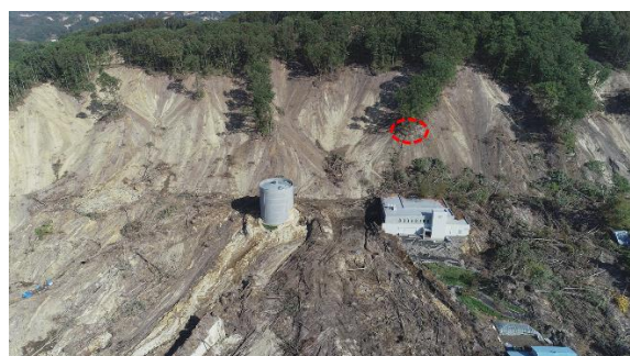
Photo 13: Location of Yanamaka Penetration test on Tomisato landslide area
