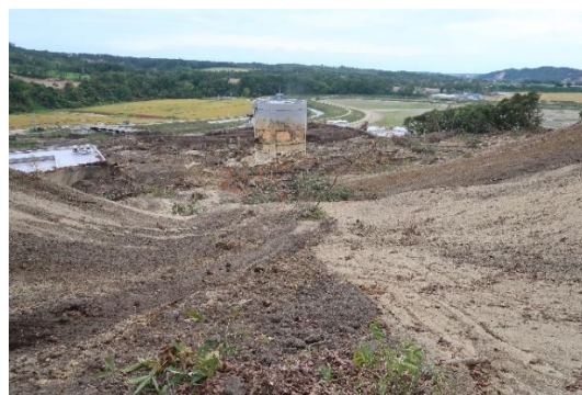
Photo 7 Downslope view of the Water tower with the imprint of landsliding debris on Tomisato area shown in Photo 6
