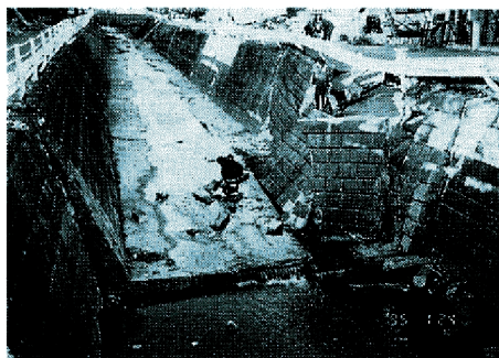
Photo 8 Collapse of concrete-block revetment of Tenjo River in Kobe
