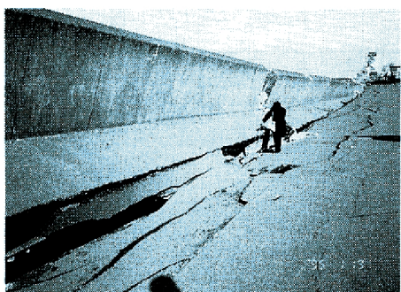
Photo 3 Top of the embankment of Yodo River
