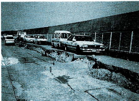
Photo 5 Damage of embankment of Kanzaki River in Osaka
