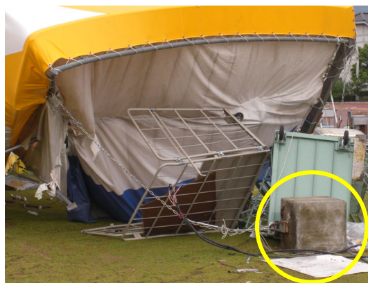
Photo 1 A concrete mass of 300kg to resist wind induces lift.
