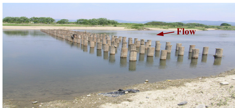
Photo 1.2 Permeable Spur Dykes along the Kizu River (May, 2005)
