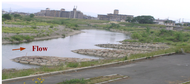
Photo 1.1 Impermeable Spur Dykes along the Katsura River (June, 2005)
