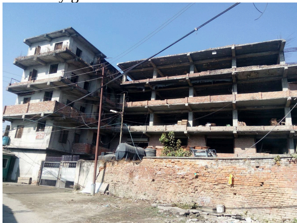
A typical industrial unit building
