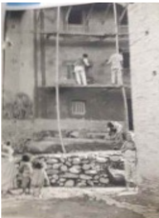
Construction/repairing work in Bungamati
