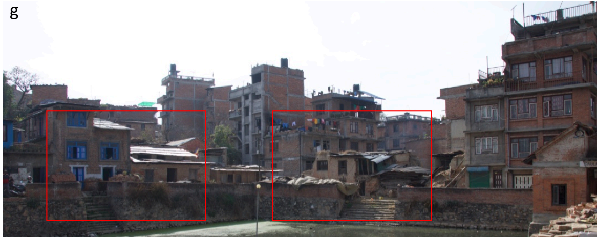
Figure 6.20 g. Photograph of the partially collapsed row houses near De-pukhu taken in 2017 with unsymmetrical openings and changes in the building materials.
