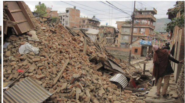
Blocking of road due to collapsed building
