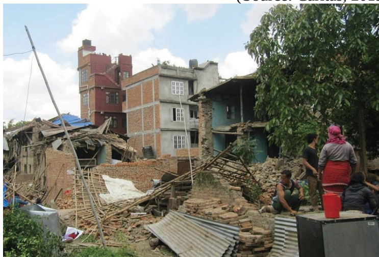
Figure 3.4 Damages to buildings in Bungamati
