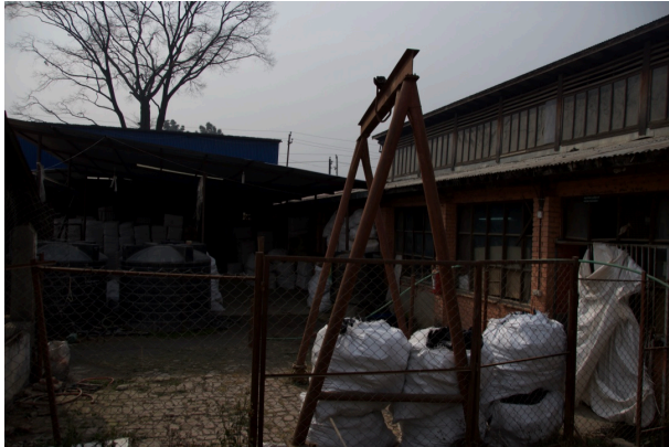
A damaged industrial building in Balaju
