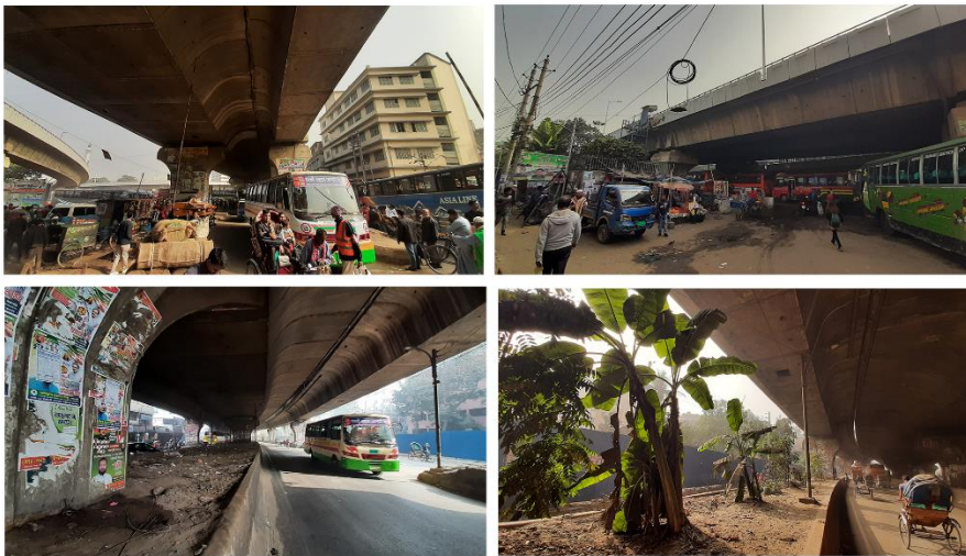
Figure 07: Mayor hanif under flyover beautification project area 01-08 (Source: DSCC,Next Door Consultant,Srijon)
