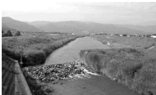
Photo 1 Rubble mound weir in Jobaru River
