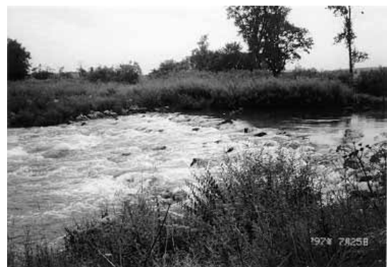
Photo 2 Rough ramp in River Danube
