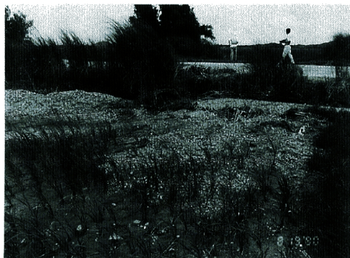
Photo 2 Liquefaction phenomenon in the vicinity of Rizal.
