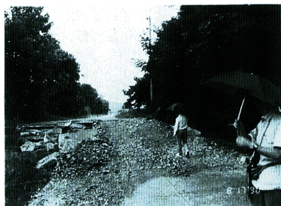
Photo 16 A surface faulting at Digdig (182 km from Manira).
