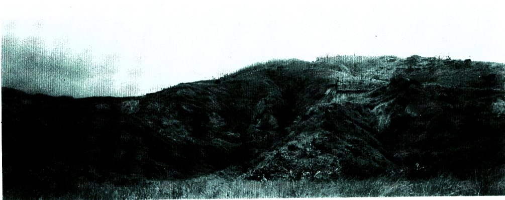
Photo 22 Slope failure ridge at Baterya.
