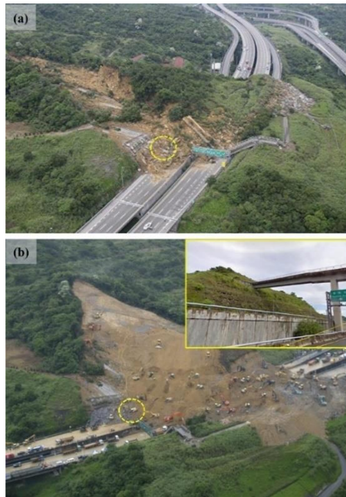
Figure 1-1 (a) Photo displaying Freeway no.3 landslide in Taiwan from NASC Taiwan (2010). (b) Photo displaying disaster relief in progress from NASC Taiwan (2010), The picture in the upper right corner of (b) is a close-up view of the pre-disaster slope, which is marked as a yellow dash circle in (a) and (b) (Yeh et al., 2021)
