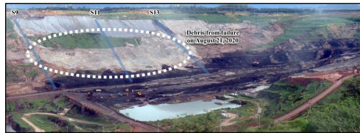
(b) Photograph of low wall failure
