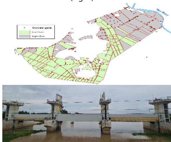
Fig. 2 Locations and a photo of the sluice gate in the field survey from July 31 to August 11, 2023
