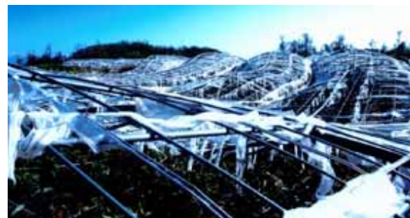
Photo 14 Damage of vinyl houses (courtesy Nougyousevenjo Miyakosijo)
