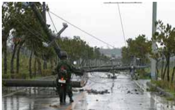
Photo 24 Broken electric poles blocked traffic (courtesy Okinawa Prefecture branch office)
