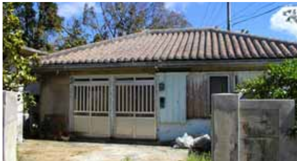
Photo 31 Traditional wooden house without damage ( Okuda et.al. 2003 )
