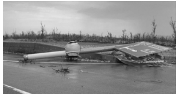
Photo 10 Break of road signs (courtesy Hirara city)
