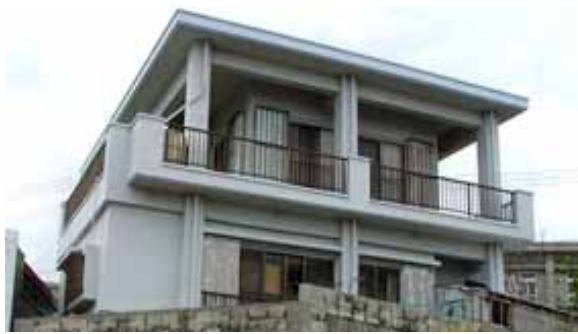
Photo 32 RC house with shutter on the windows
