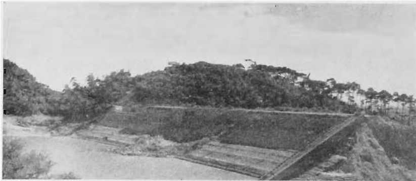
Photo. 5 Failed Aiai-ike Dam (left: spillway, right: drain holes with sluice gates).
