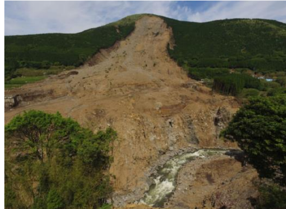
Fig.1 The front view of Aso Bridge landslide
