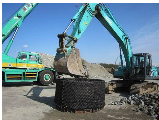
Photo 2 Filling of inner rubble
