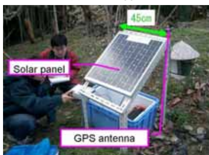
(c) solar panel
