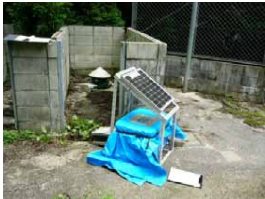
(c) on concrete floor
