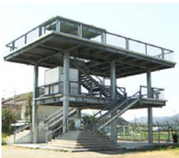
Fig 2. Current Tsunami Evacuation Tower
