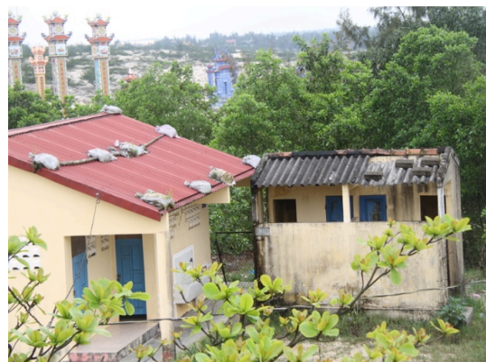
Typhoon mitigation by using sand bag to secure the roof
