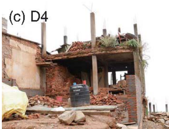
Fig. 4 Photo of buildings with damage levels D2-D4. (a) D2: plasters on the column was fallen down. (b) D3: permanent drift was observed. (c) D4: almost all infil was fallen down.
