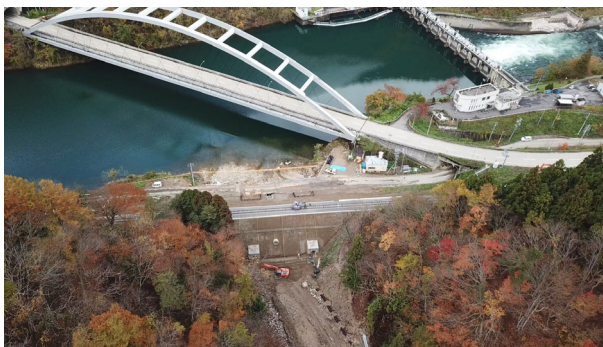
Fig. 3 Uchiho Dam Reservoir where debris flows flowed into.
