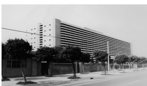
Fig.2-24 Chingling Industrial Research Center
