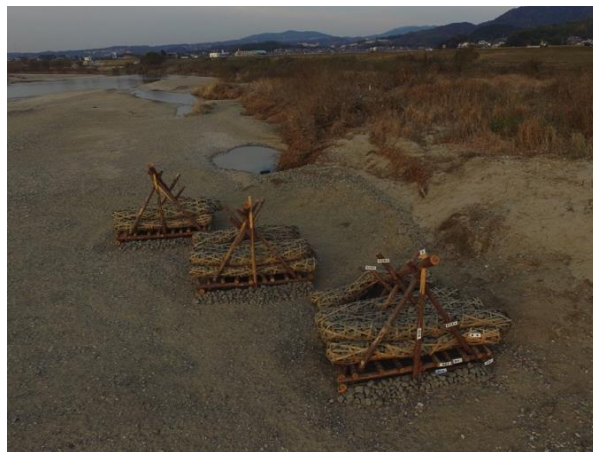
Photo 1 “Seigyū” (crib spur) set up in the Kizu River as a test trial in December 2017
