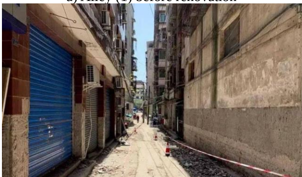
c) Alley (2) before renovation
