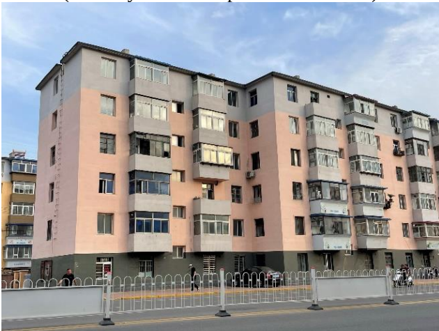
(c) Vacant Residential Building
