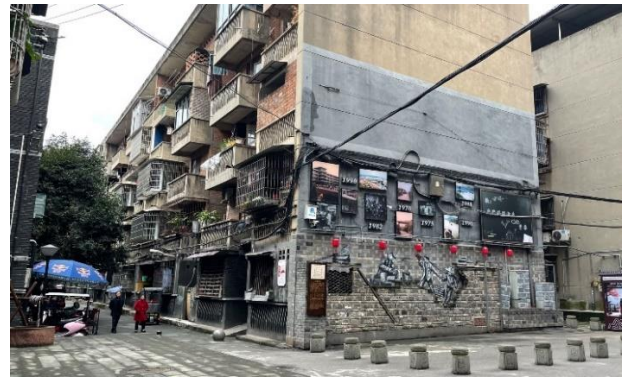
b) Inconsistent building facades
