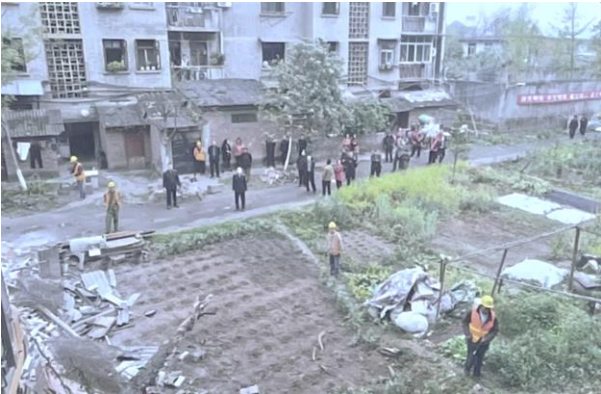
a) Demolition of illegal structures (location 1)
