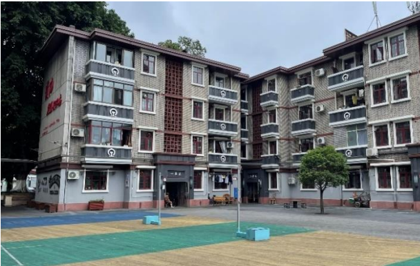
b) Renovated into a community square (location 1)
