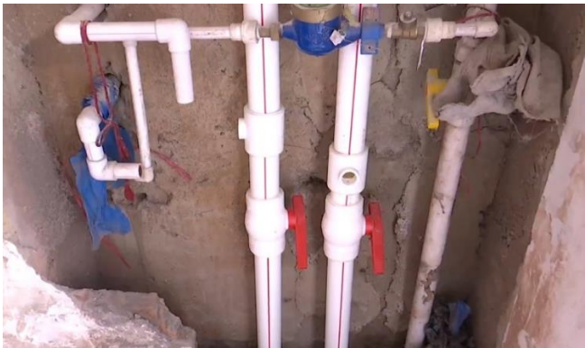
b) Water pipeline renovation
