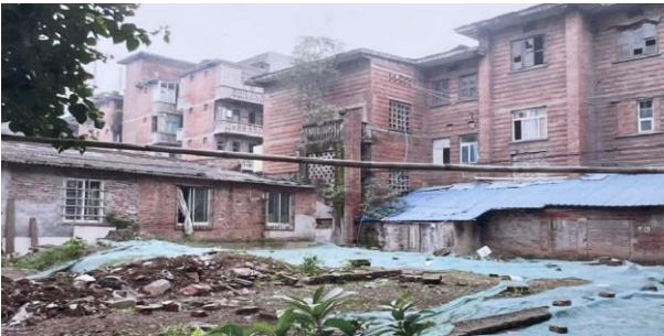
e) Demolition of illegal structures (location 3)
