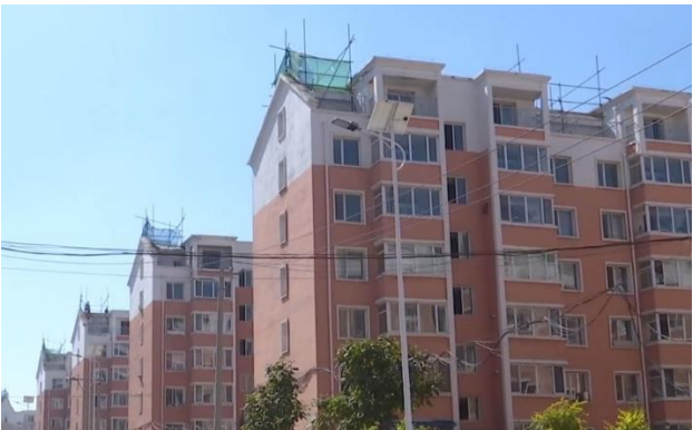
a) Roof waterproofing renovation
