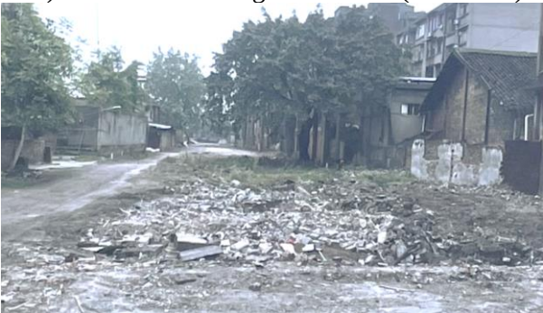
c) Demolition of illegal structures (location 2)
