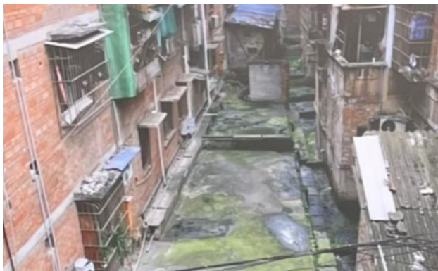
a) Alley (1) before renovation
