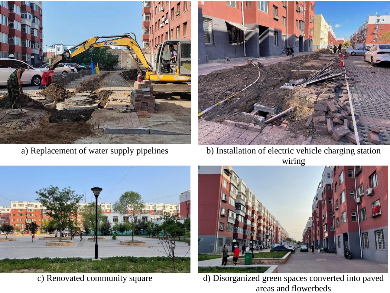
Figure 5.4 Scenes During and After the Renovation (WXY)
