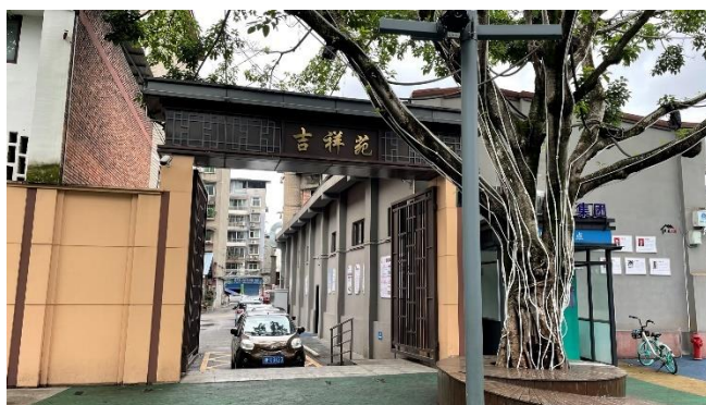
a) This is the gate on the south side of the main square. There is a height difference between the inside and outside of the gate, causing rainwater to flow towards the buildings on the inner side.
