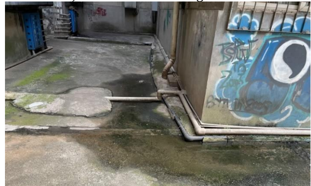
d) Exposed pipes
