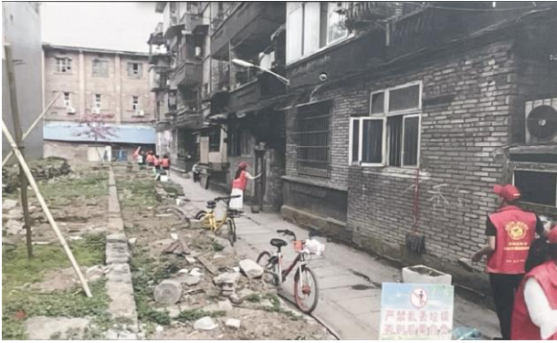
g) Demolition of illegal structures (location 4)
