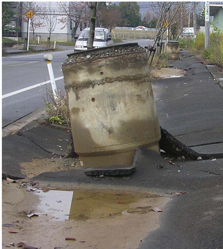
Fig. 1.1 Uplifted manholes and settlements of sidewalk after the 2004 Niigata-ken Chuetsu, Japan, earthquake.
