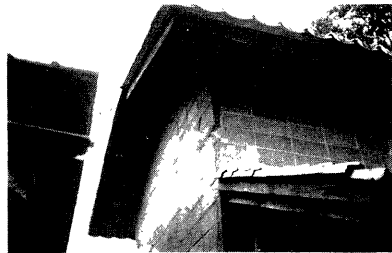
Photo 4 Cracks in concrete block wall
