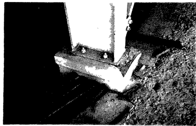
Photo 6 Damage at column base
