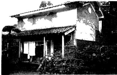
Photo 1 Falling down of wall finishing
