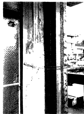
Photo 12 Shear failure of a reinforced concrete column
