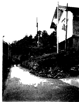
Photo 2 Failure of banking soil
