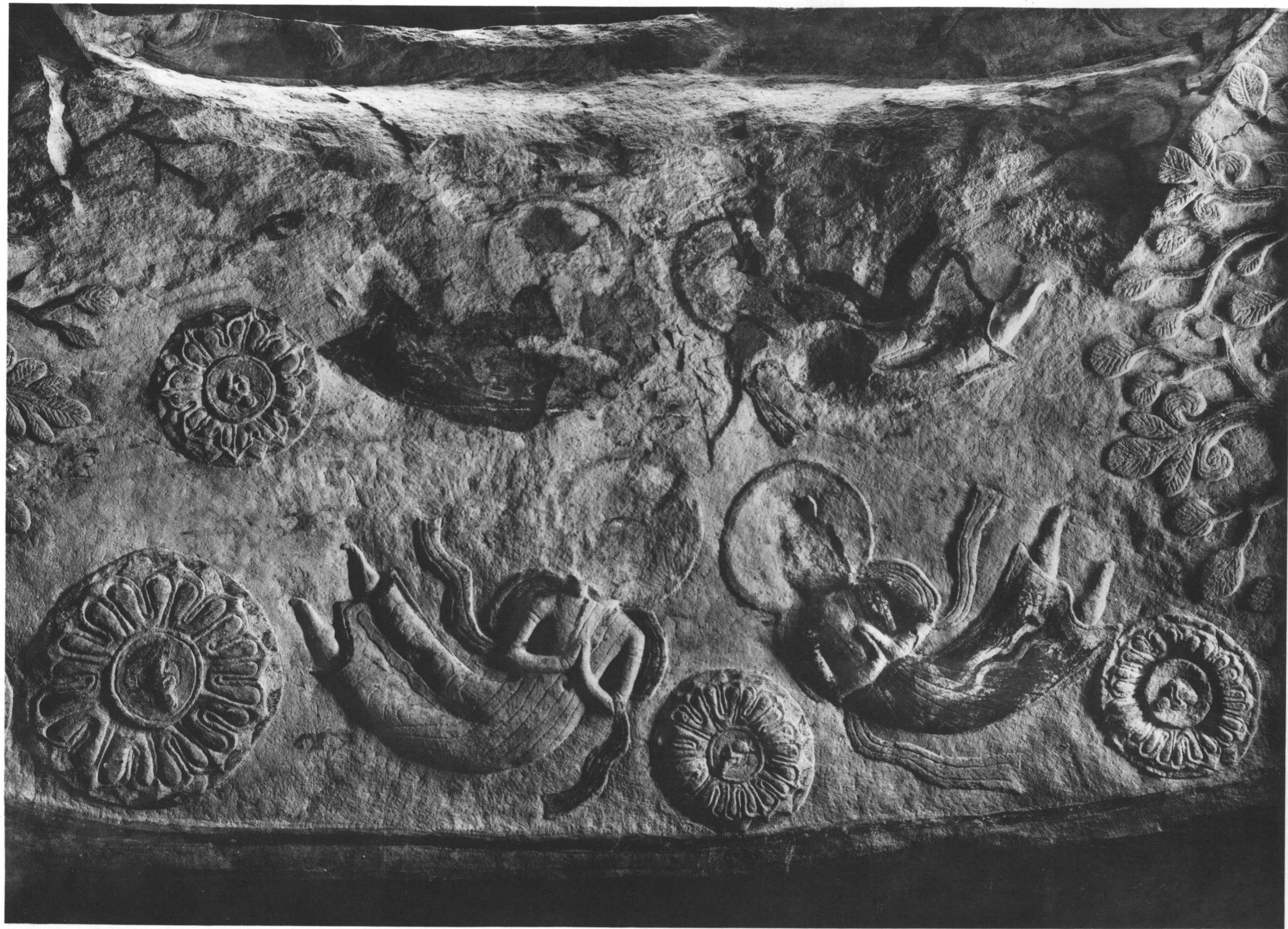
Entrance Gateway, Ceiling.
