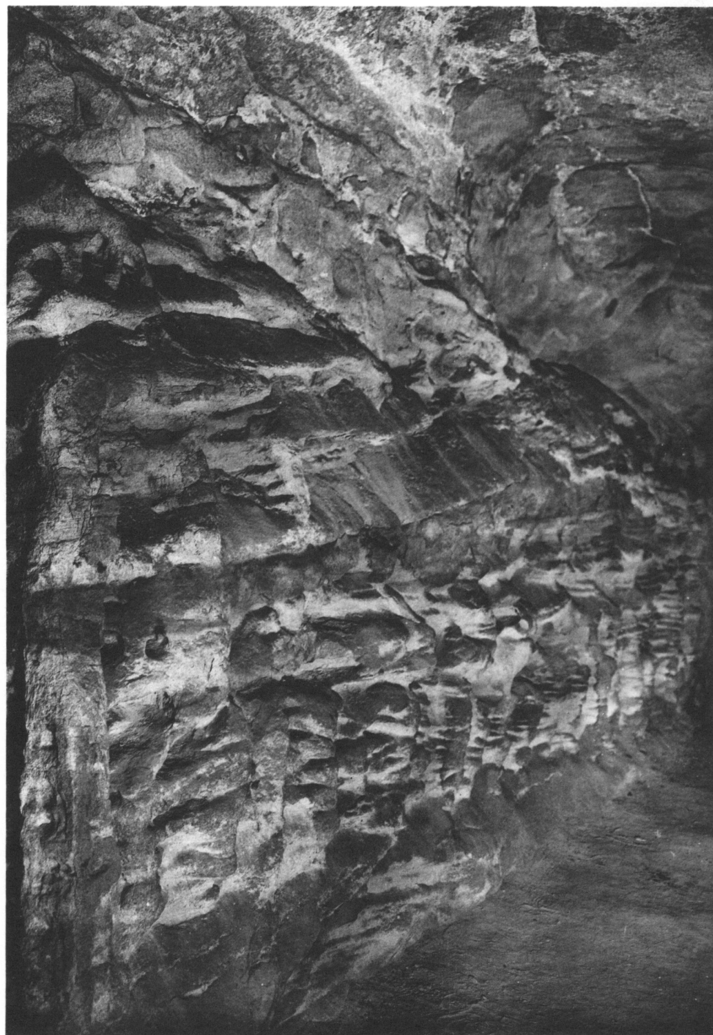
A) Passage, South Wall. 隧道 南壁
