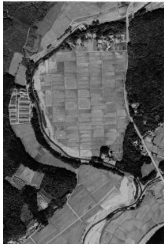
Photo 10 Aerial photograph taken after the flood around the junction with the Sanzogawa River
