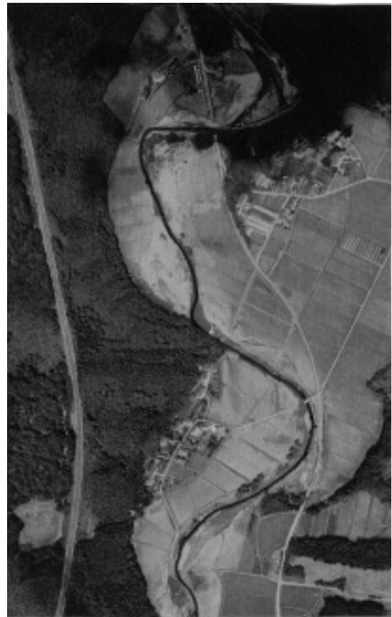
Photo 6 Aerial photograph taken after the flood around the Kurokawa bridge and Yajiro bridge
