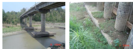
Photo 10 Effects of riverbed degradation by excess sand mining on river structures in Indonesian rivers
