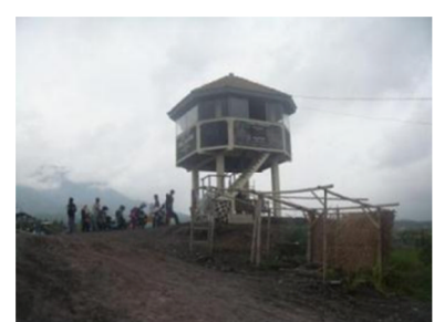
Photo 12 Monitoring tower by NGO in Gendol River
