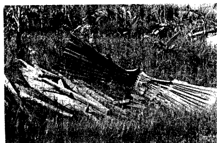
Photo. 3 Blown-away and crashed tin roof of a garage, Ozato, OKINAWA.
