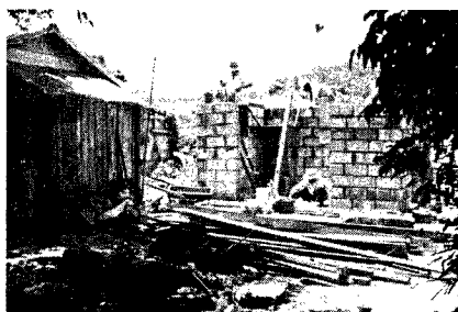
Photo. 2 Inclined concrete block walls of a house, Zaha, OKINAWA.
