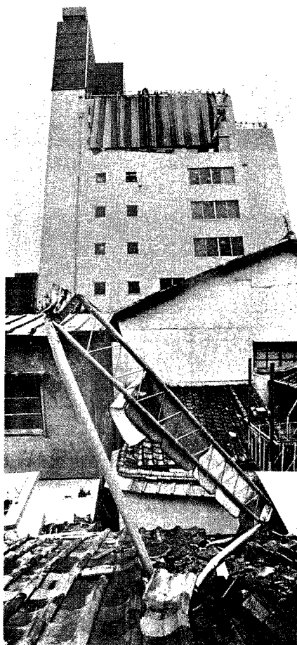
Photo. 12 Tent frame blown-away from the top of a 8-streyyed building, KYOTO (by the courtesy of the Kyoto Shimbun).
