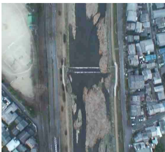
Photo 6 The aerial photo of the upper of the Kamigamo Bridge
