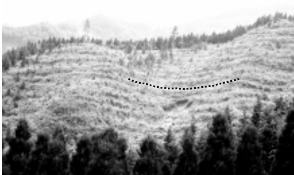
Photo 6 Collapse in natural slope A
