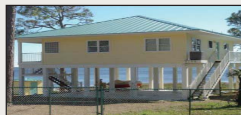
Figure 8: Raised houses in flood-prone areas: Japan (top left), Bangladesh (top right), and USA (bottom right). From DRH 8, 16, and 17
