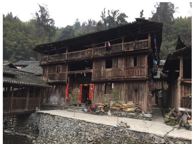
(b) Typical residential buildings
