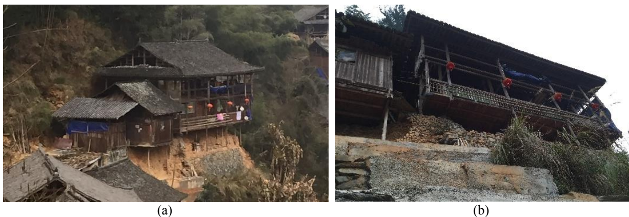
(a) The most severely affected building, whose foundations have already collapsed (b) This household was repeatedly repairing and strengthening the foundations with stone and cement
