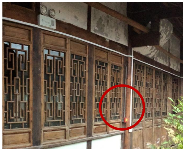
Figure 7.7 Fire alarm only assembled in the most important heritage building in Shangli Village
