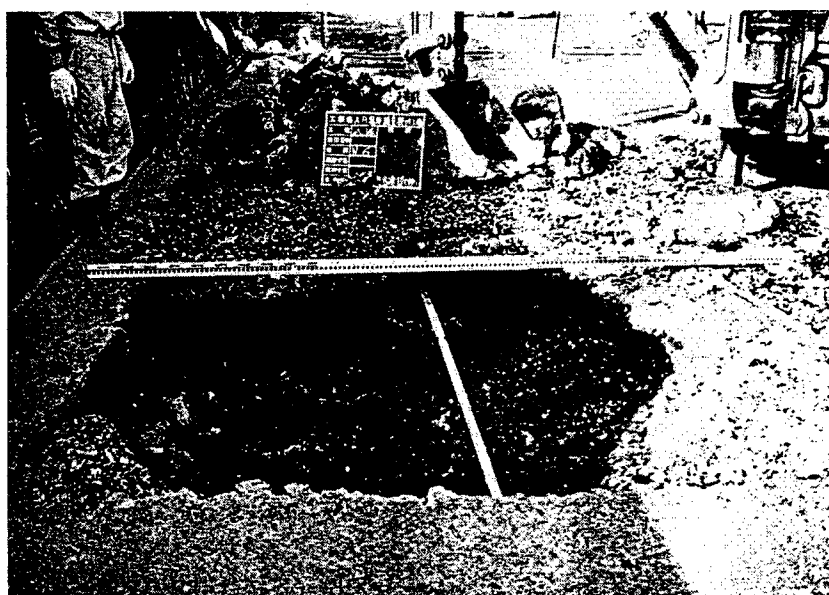
Photo. 1 Cavitation under the pavement behind revetment.
