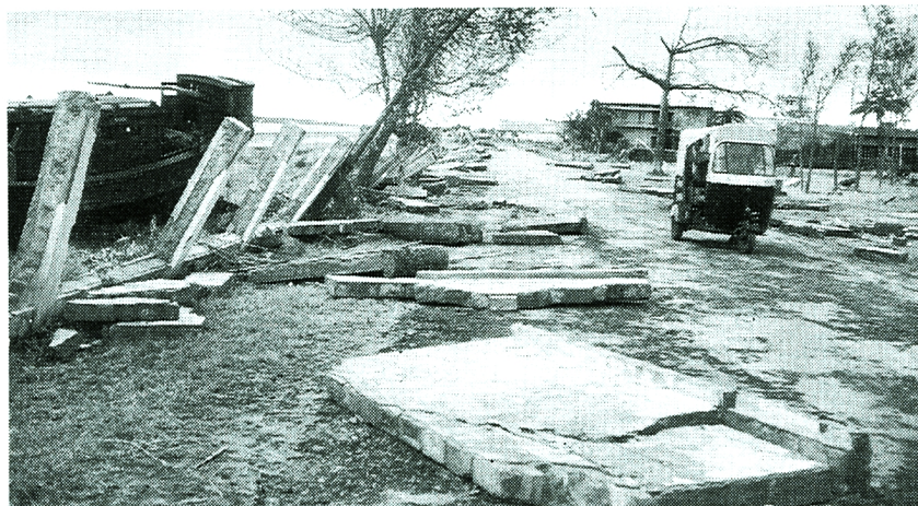
Photo 6. Brick wall toppled by flooding water.
