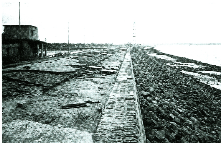
Photo 7. Damaged levee that had been armored with asphalt and bricks along the right side of the mouth of the Karnafuli River.
