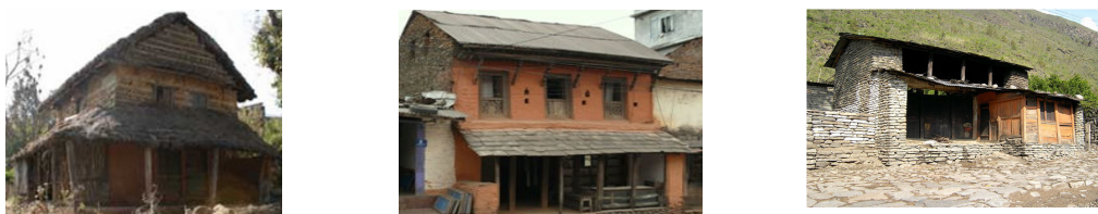
Fig.6.1 Typical stone masonry houses in Nepal
