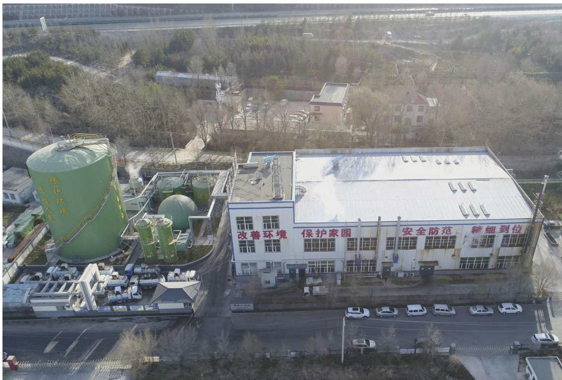
Figure A.4. Working biogas plant in China
