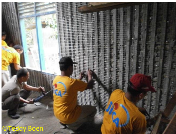
Trained Local Masons Stitching the Inside and Outside Wire Mesh
