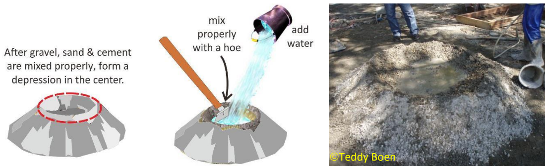
Figure 32 – Preparing Concrete Mix
