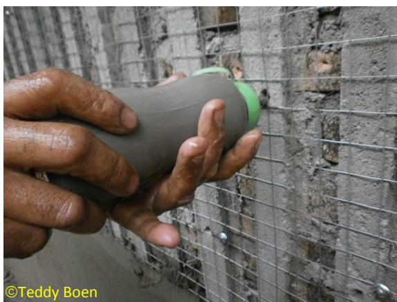
Grouting of Drill Holes using Cement Paste
