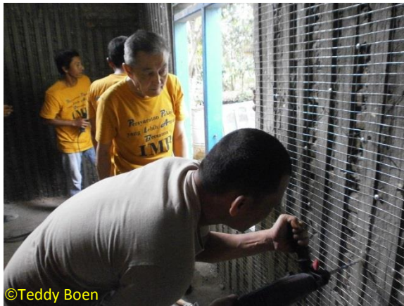
Drilling the Walls for Stitching
