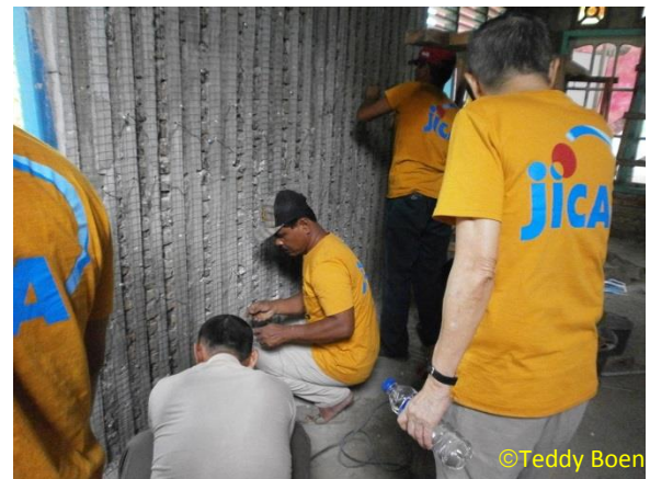
Trained Local Masons Stitching the Inside and Outside Wire Mesh
