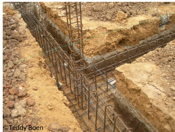
Figure 31 – Reinforced Concrete Inverted-T Foundation
