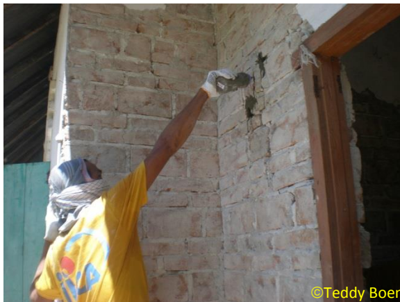
Sealing the Cracks with Cement - Sand Mortar
