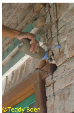
Figure 90 – Cracks are sealed with Cement - Sand Mortar; Walls are sprayed with Cement-Water
