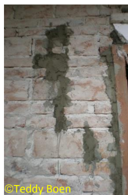
Figure 90 – Cracks are sealed with Cement - Sand Mortar; Walls are sprayed with Cement-Water
