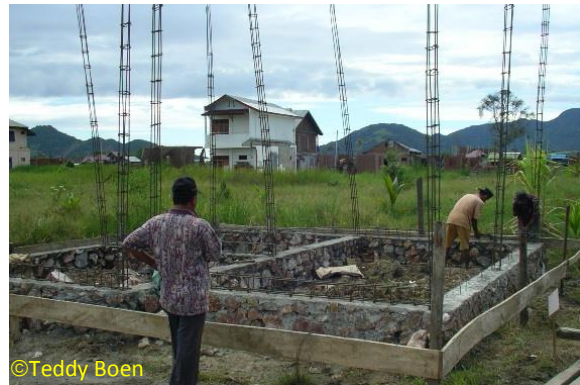
Figure 30 – Rubble Stone Foundation
