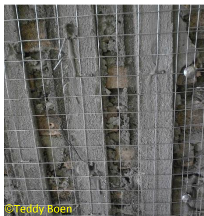
Figure 97 – Grouting of Drill Holes Using Cement Paste
