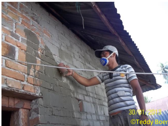
Spraying Walls with Cement-Water
