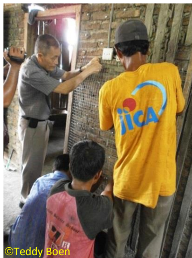
Installation of Wire Mesh, Tie to Umbrella-Head-Roofing-Nail
