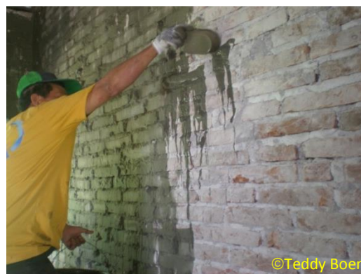
Figure 90 – Cracks are sealed with Cement - Sand Mortar; Walls are sprayed with Cement-Water
