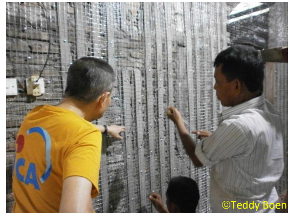
Stitching the Inside and Outside Wire Mesh
