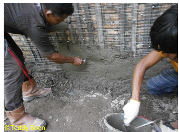
Re-plastering the Wall
