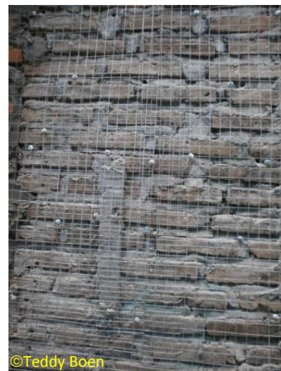
Wire Mesh Installed and Fastened to Top of Umbrella-Head-Roofing-Nail
