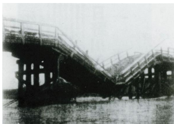
Photo 4 The Ichido Bridge was damaged by Typhoon Isewan (source: Shiga Prefecture homepage)
