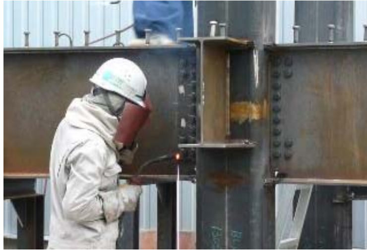
Figure 5.4 Vertical welding in web
