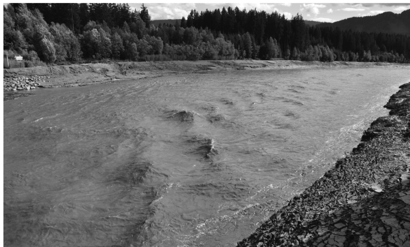
Figure 2.21 Standing waves during the flushing operation of 2012 observed upstream of the weir (Harb et al., 2014).
