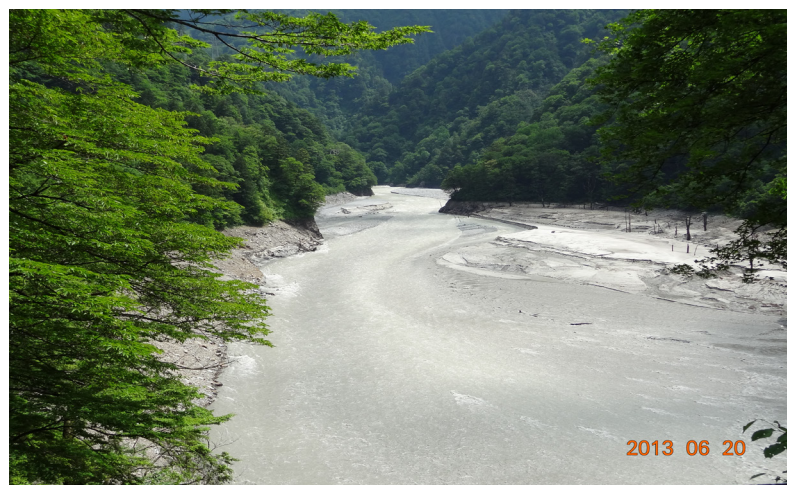
Figure 2.11 Shallow flow condition during the free-flow stage of flushing operation at the middle reach of Dashidaira reservoir (Photo taken by author).
